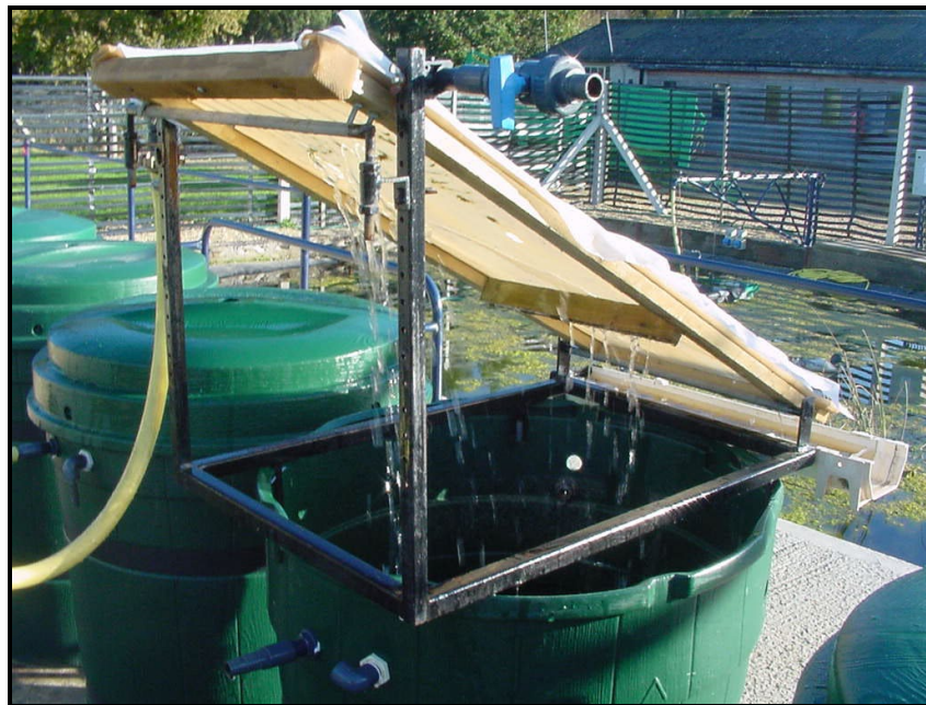
Figure 8: Run-down separator in operation with a 50 \mu\text{m} filter mesh showing the effect of placing a small baffle on the under surface of the mesh in directing the filtered water to the top of the SSF.
