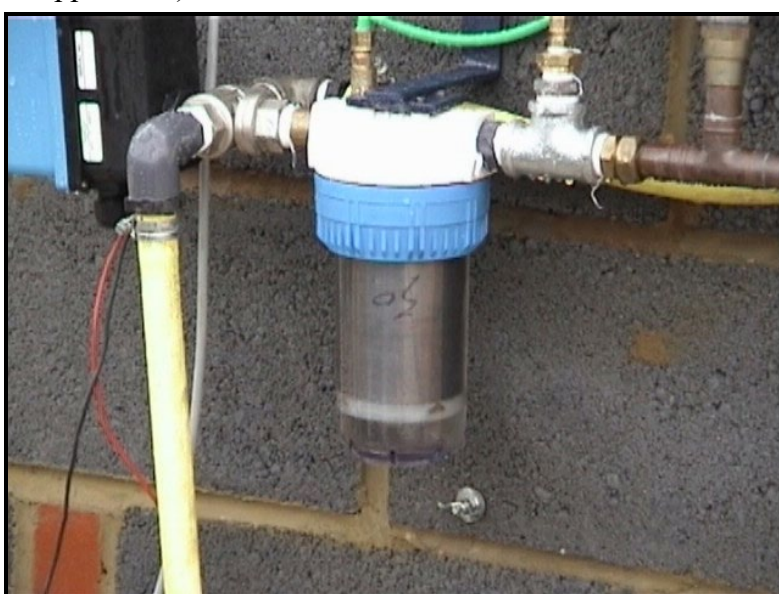
Figure 3: Close-up photograph of the Cross EasyClean filter set up with a 50 \mu\text{m} filtration cartridge (for details of this pre-filtration system see Appendix I).
